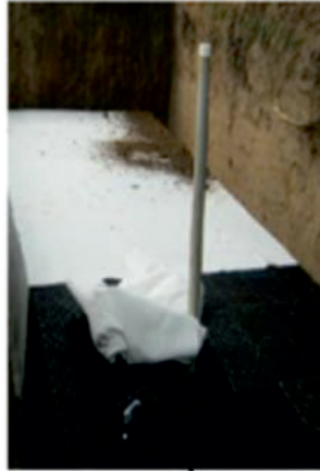
7 Module being wrapped with Geotextile
