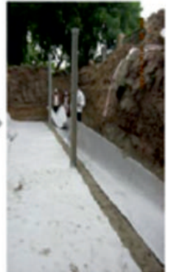
8 Module wrapped in Geotextile
