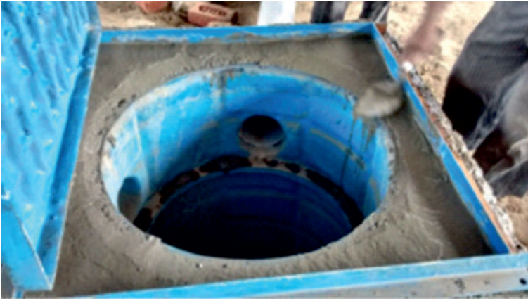
FRP (or similar materials) Tank with micro-filter (Geotextile)
