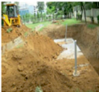
9 Backfilling port installation
